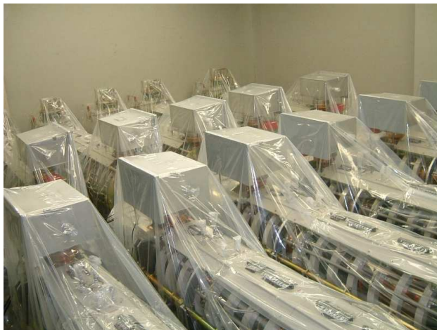
Klystrons, a circulator and wave guides
