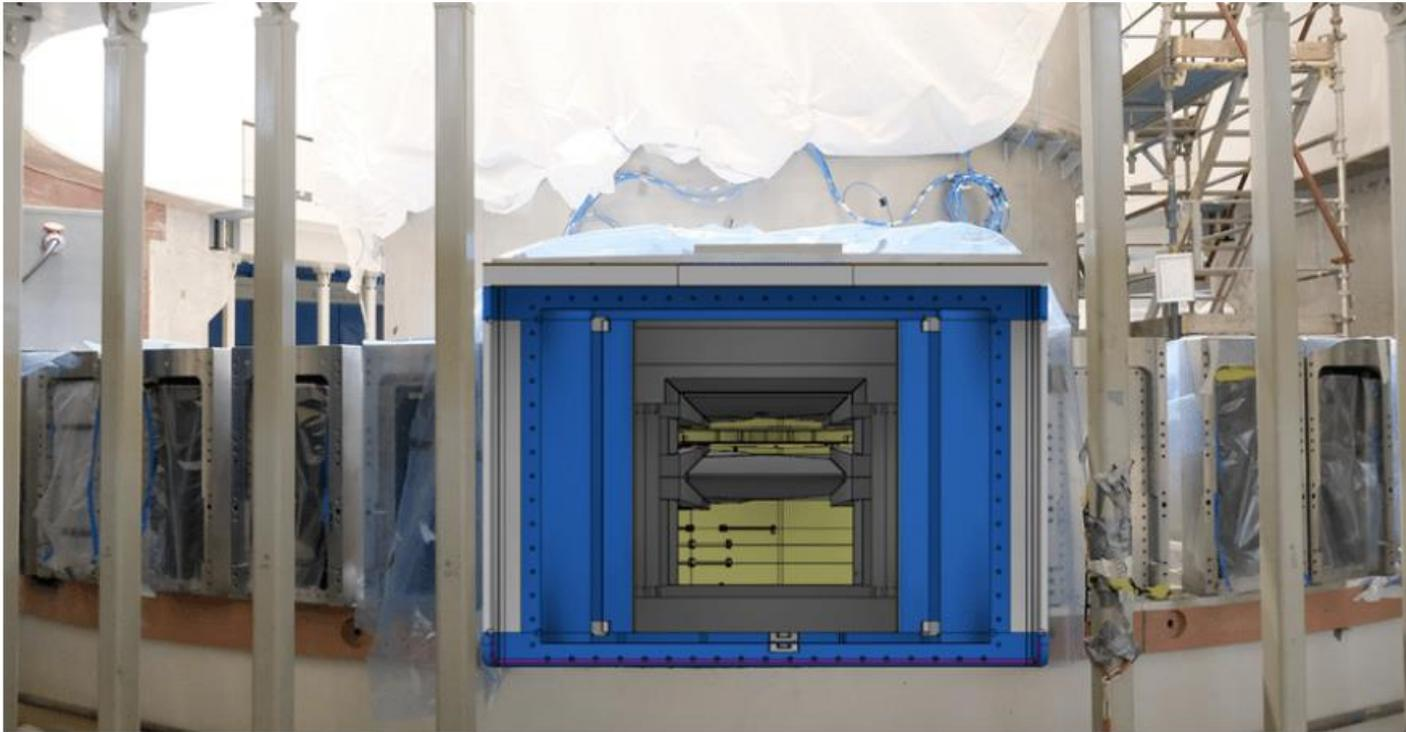
Photograph of the frame of the Large Beam Port being installed in the ESS monolith. A superimposed CAD drawing is showing the field of view of the LBP. The upper moderator, the inner shielding to avoid a direct view of the target, and the space below the target where the high-intensity moderator will be placed, can be clearly seen.
